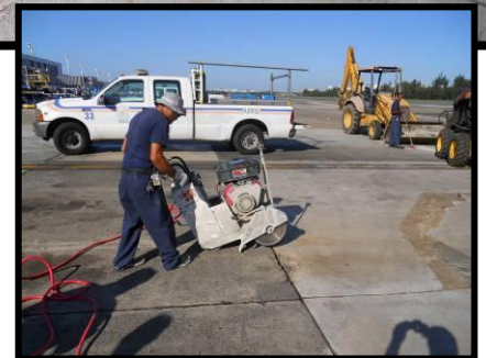
AIRPORT SPALL REPAIRS
