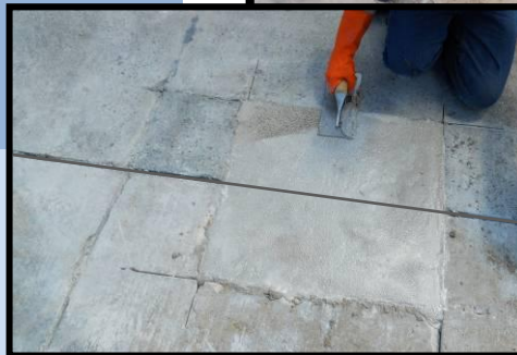
AIRPORT SPALL REPAIRS
