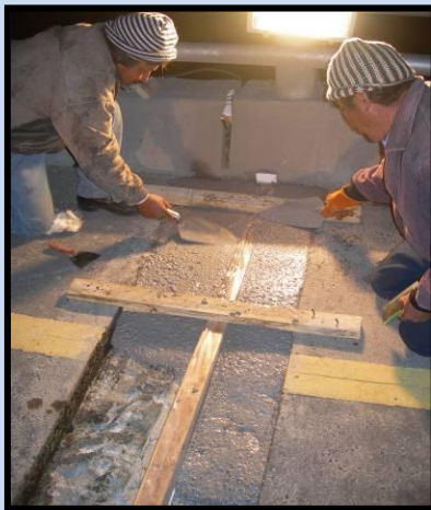
JOINT REPAIRS
